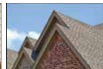
Roof Replacement & Insurance Claims
