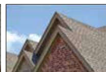
Roof Replacement & Insurance Claims
